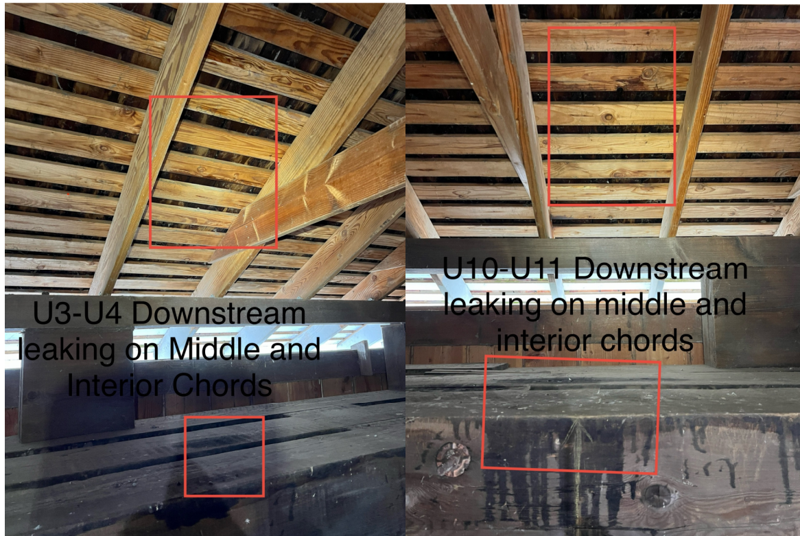
Leaks in Roof over Downstream Top Chord
