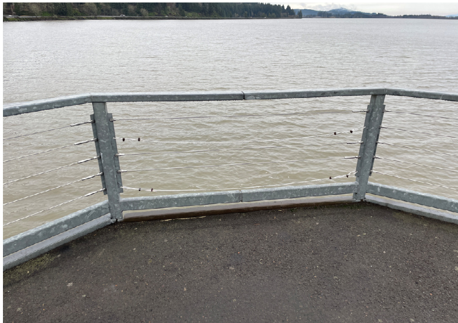
Span 4 Outlook Cable Handrail
