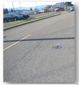
Longitudinal and Transverse cracks are usually caused by environmental impacts (freeze and thaw), swelling or shrinkage of the subgrade, poor construction methods,
