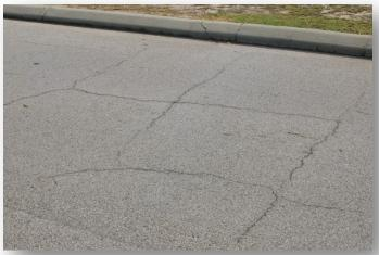
Figure 3-4 Block Cracking (not in Lowell)
