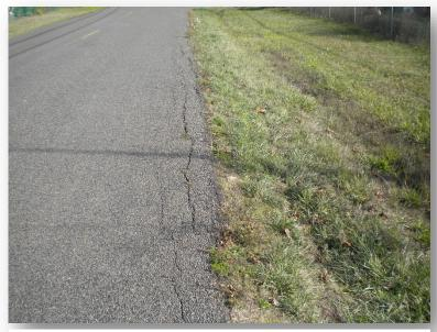
Figure 3-2 Edge Cracking on 2<sup>nd</sup> St.
