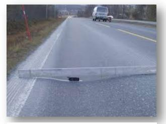
Figure 3-6 Pavement Rutting (not in Lowell)
