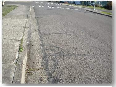
Figure 3-1 Alligator Cracking on Main St.
