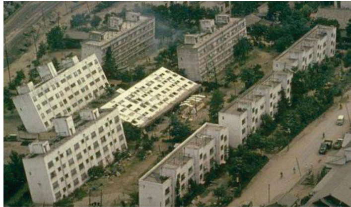
Liquefaction during the 1964 Niigata M7.6 earthquake, Honshu, Japan caused major foundation failure in these apartment blocks. Image from WikiCommons.
