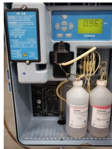
PHOTO 7.2.2 – CHLORINE ANALYZER
