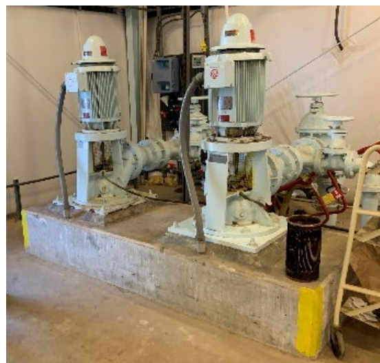
PHOTO 7.2.3 – FINISHED WATER PUMPS
