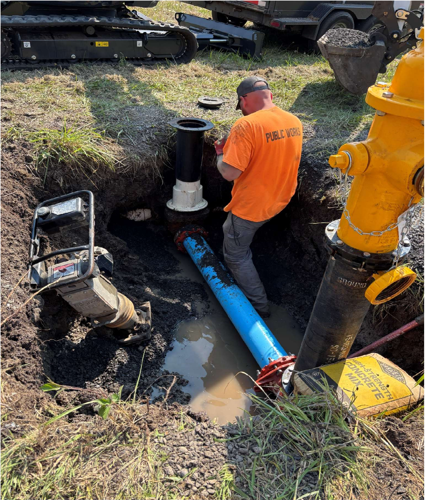
Fixing Fire Hydrant - Photo Courtesy of Public Works
